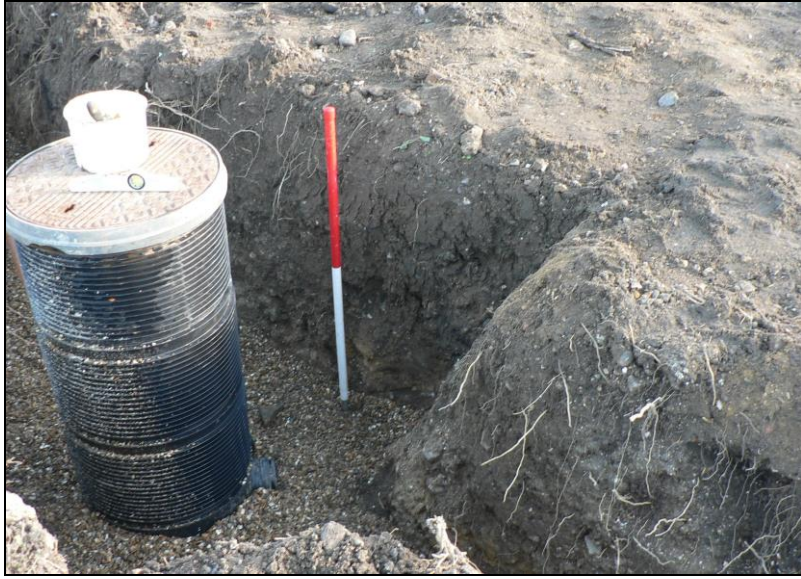
Drainage trench in southern central part of the site
