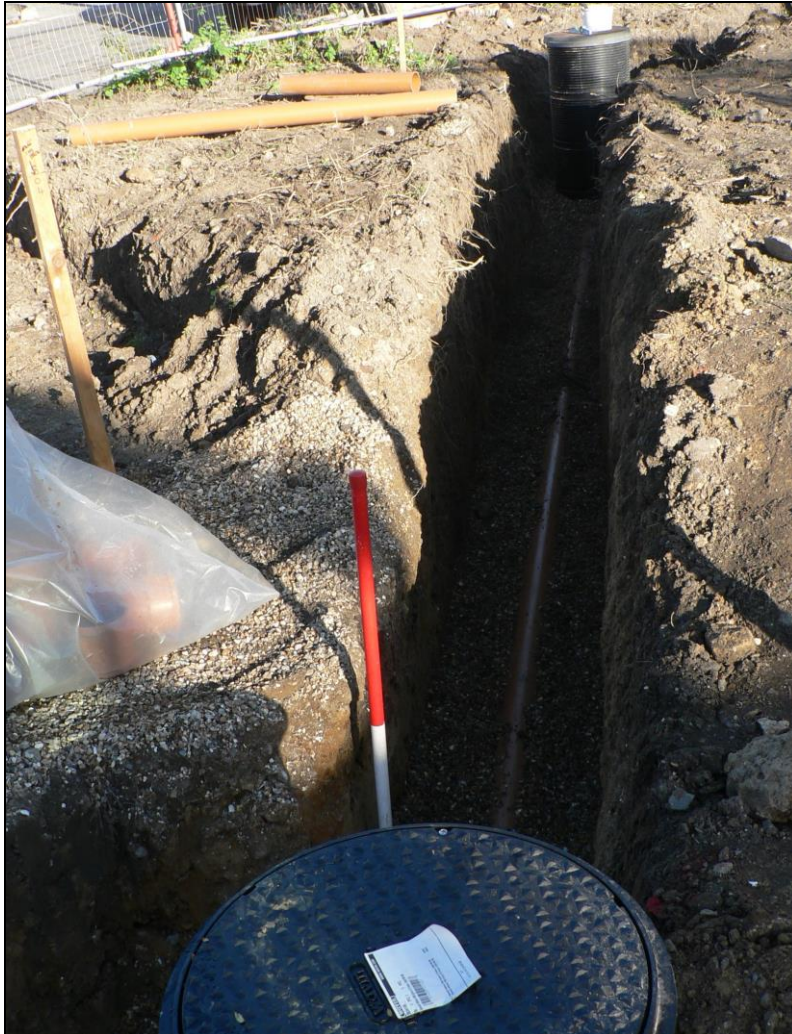
Drainage trench in north-eastern part of the site
