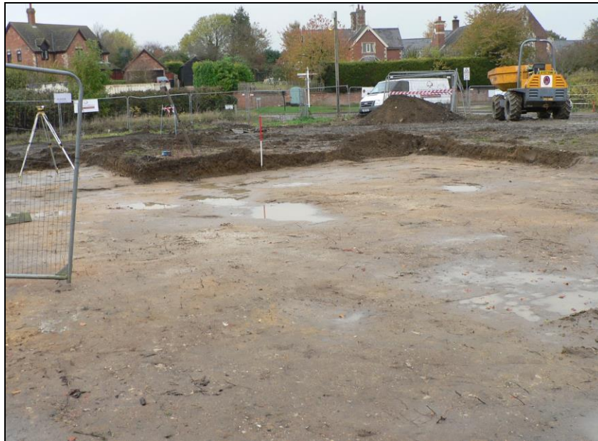
Soil strip for north-western dwelling plot
