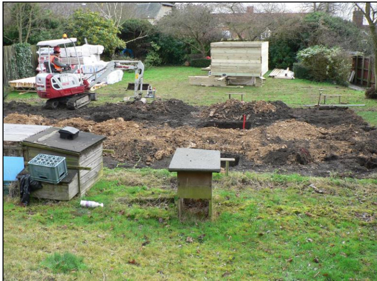
General view from north
