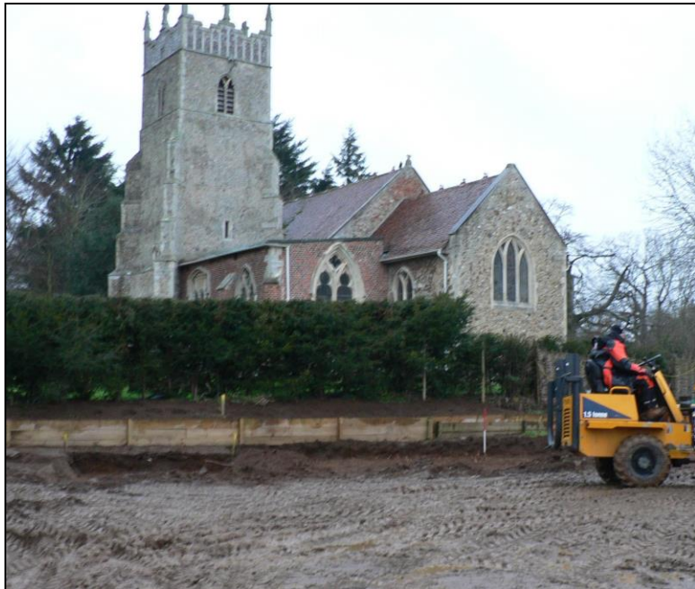
General view from west during soil strip
