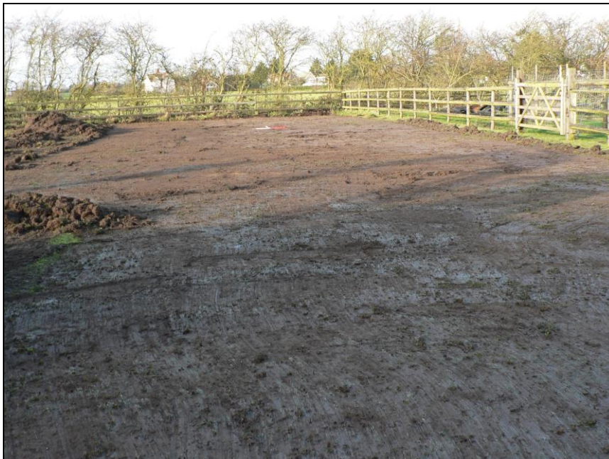
General view from east during soil strip
