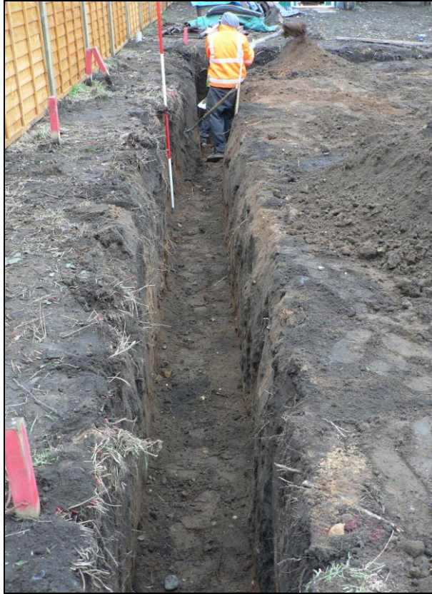
Southern trench from east
