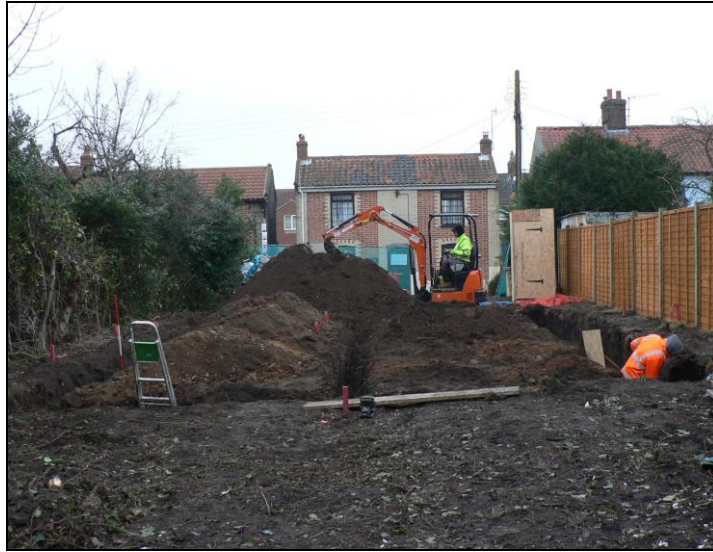
General view from south-west
