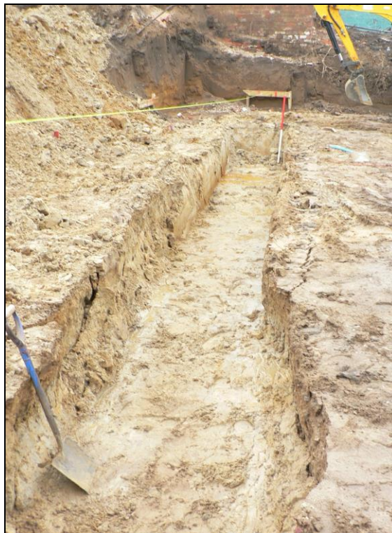
Foundation trench for plot 4 from east
