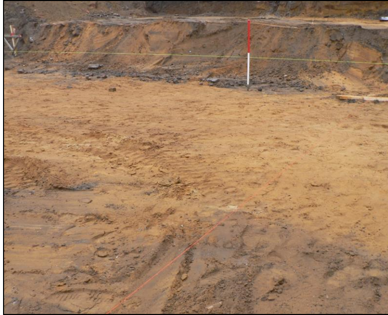
Stripped area for plot 3
