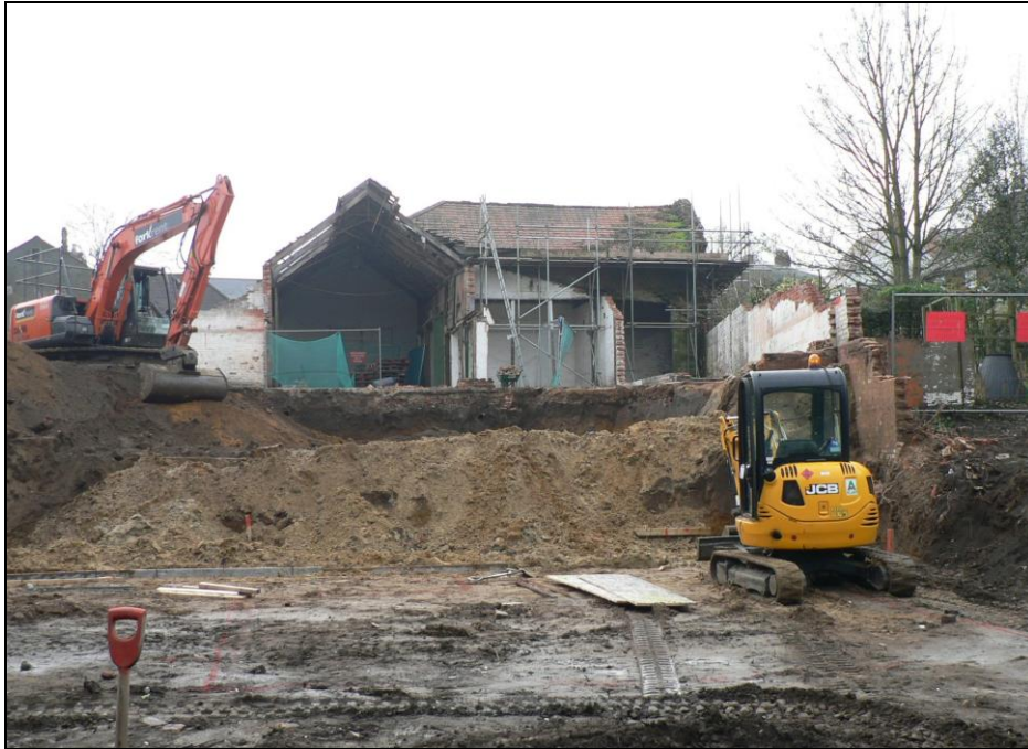
General view from north during ground reduction
