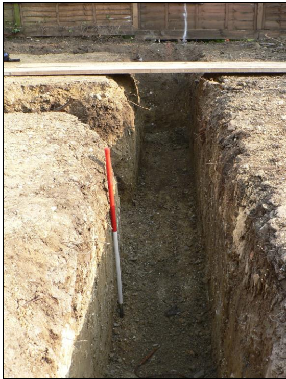
Foundation trench on western side from north
