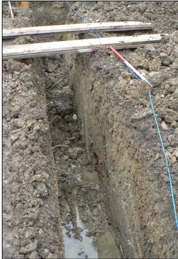
Eastern foundation trench from south
