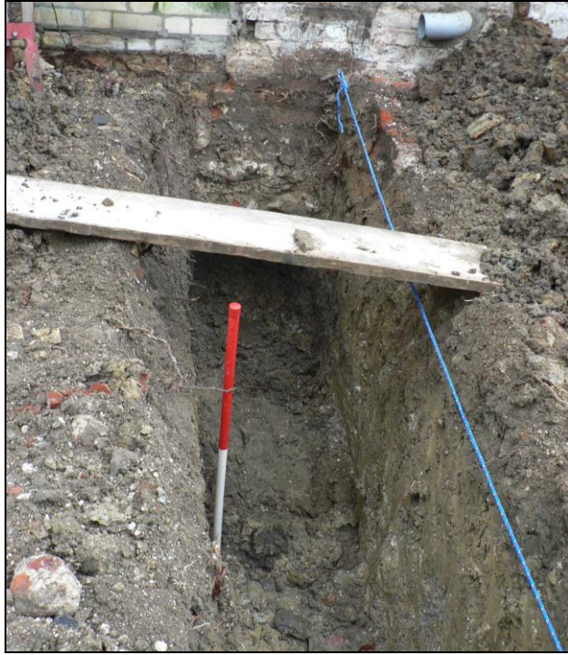
Northern trench from east
