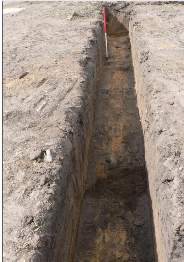
Southern trench of southern plot from east
