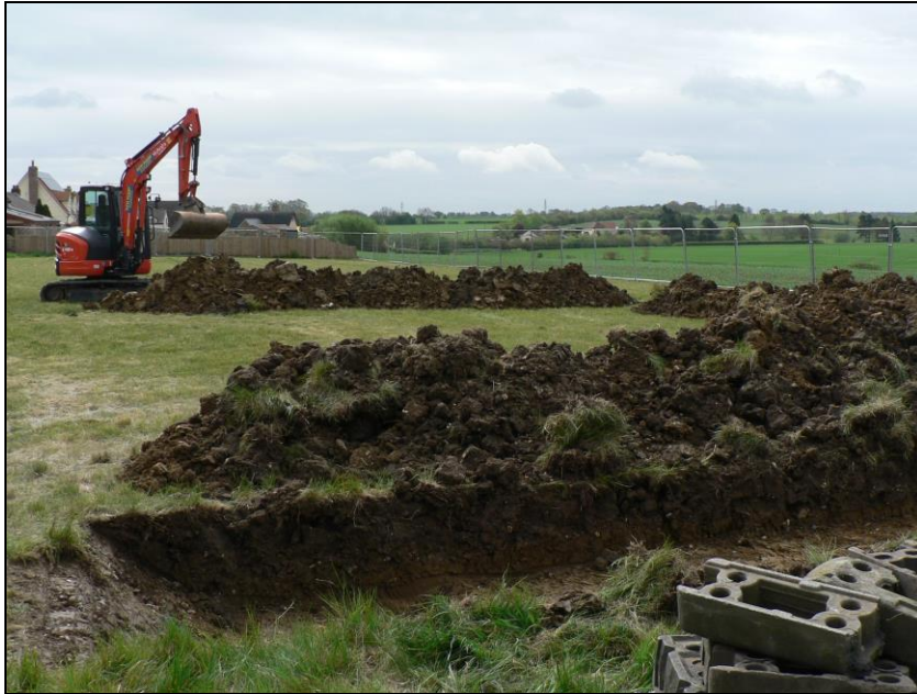
General view from north
