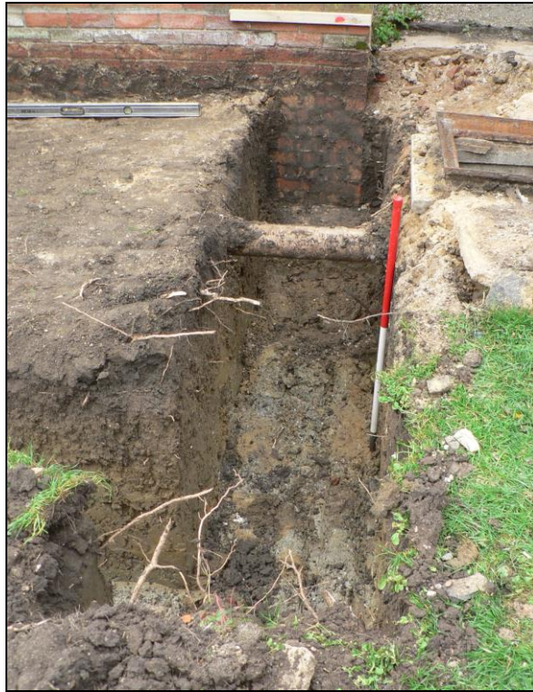
Western trench from north
