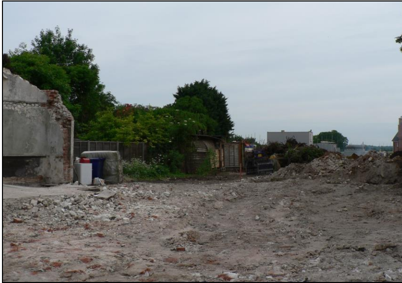
General view from west
