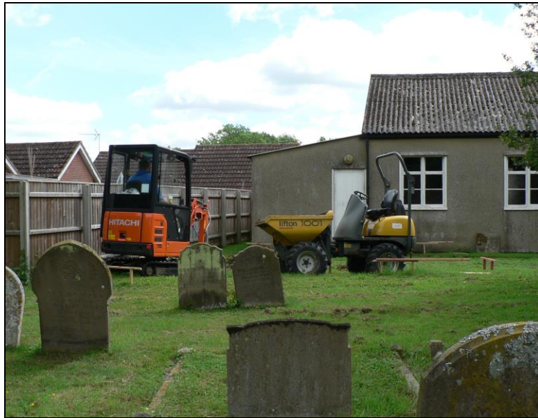
General view from west
