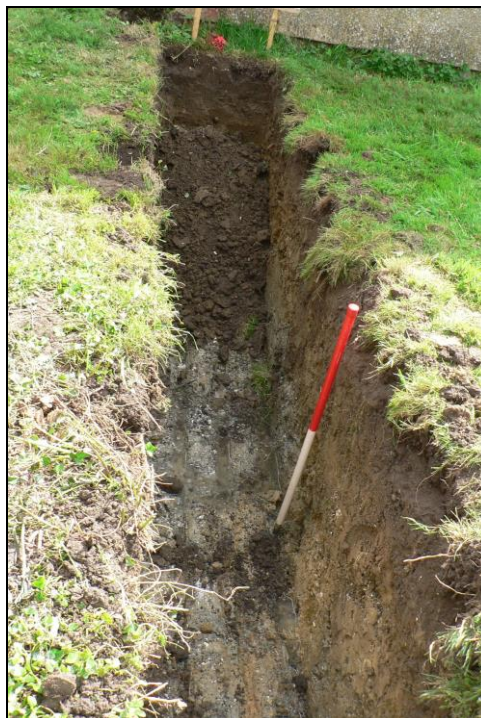
Northern trench from west
