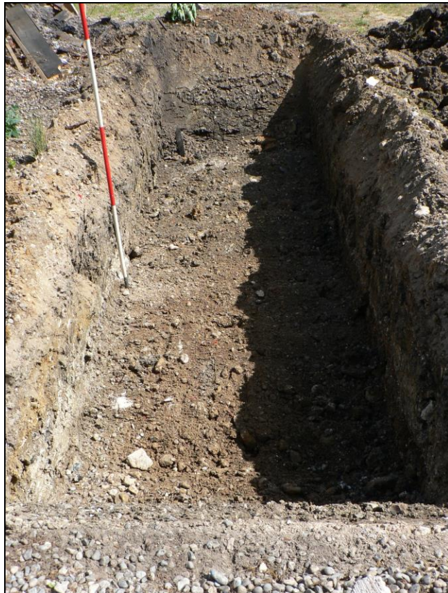
Trench 10 from south
