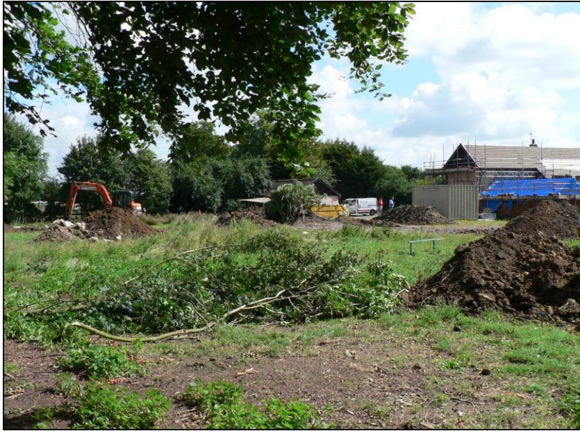
General view from southwest
