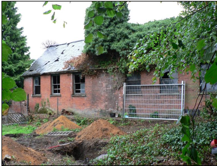
General view of outbuilding from southeast
