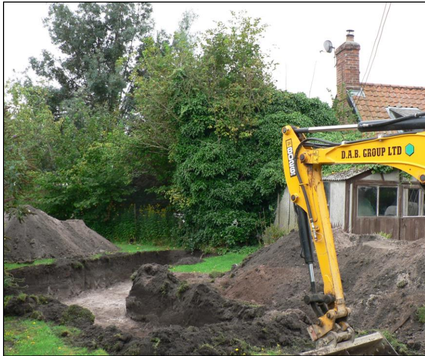
General view from north
