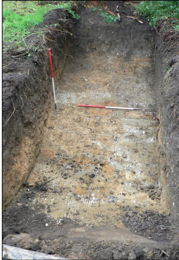
Trench 2 from west
