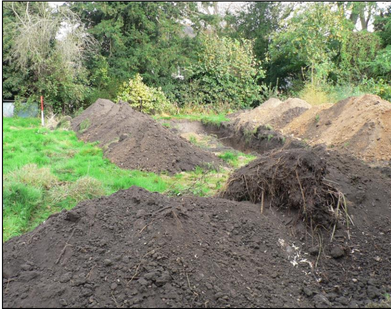
General view from southwest
