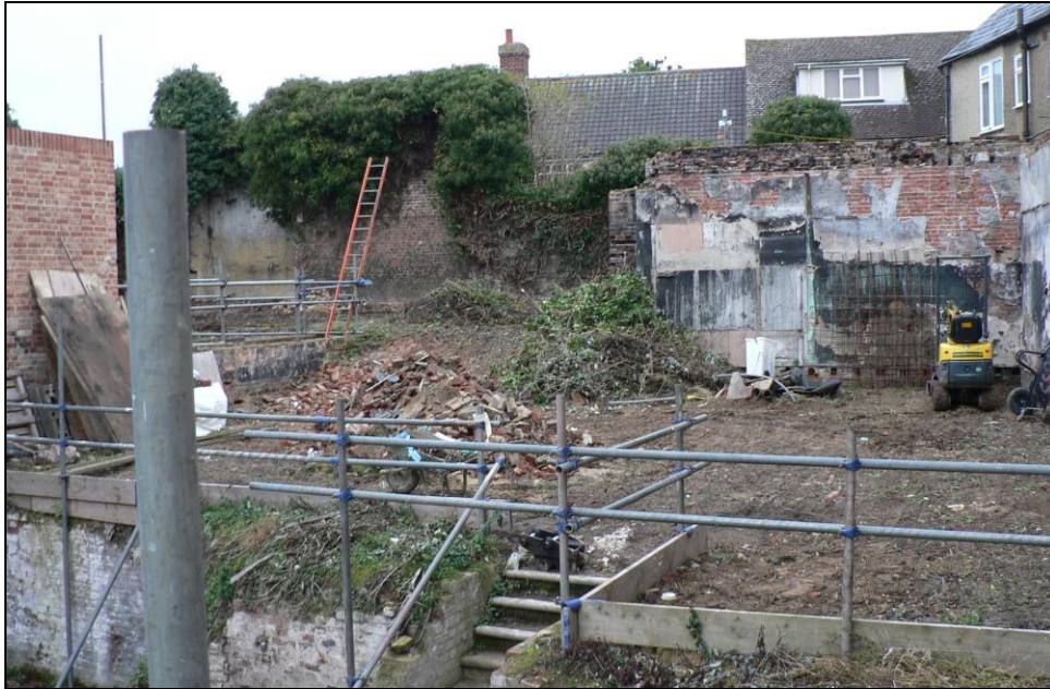
General view from Friars Street
