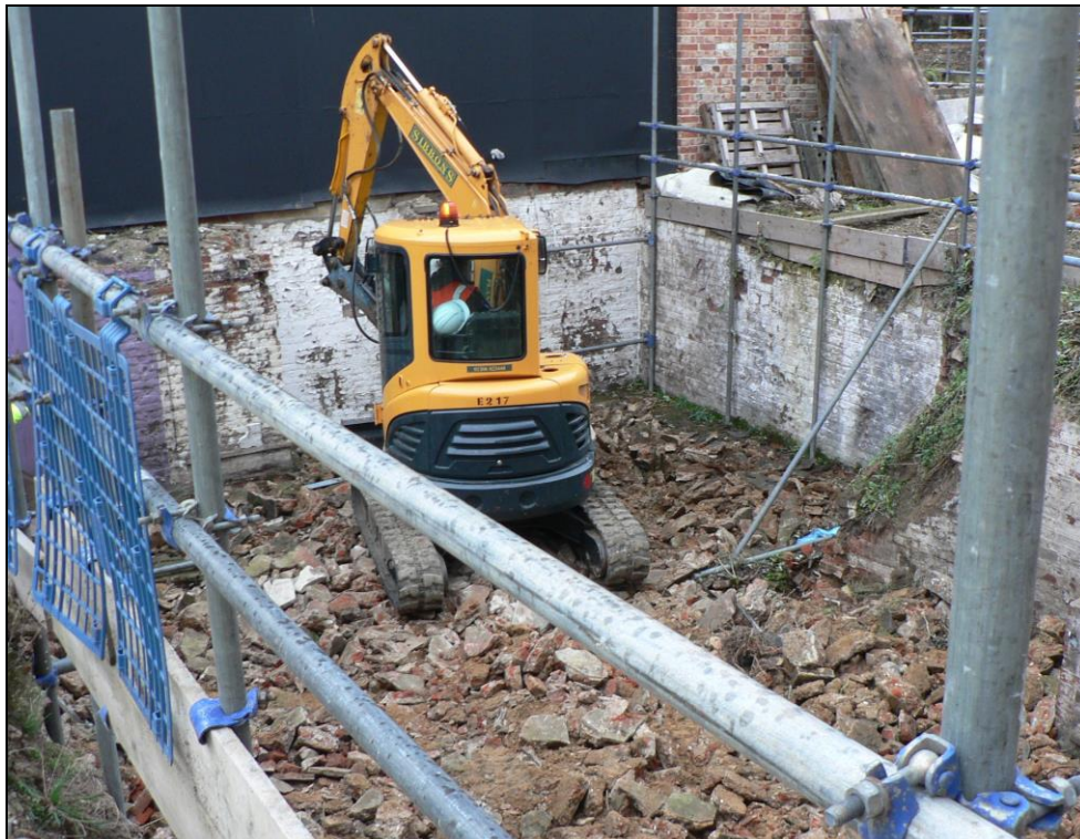
Breaking out cellar floor on Friars Street frontage
