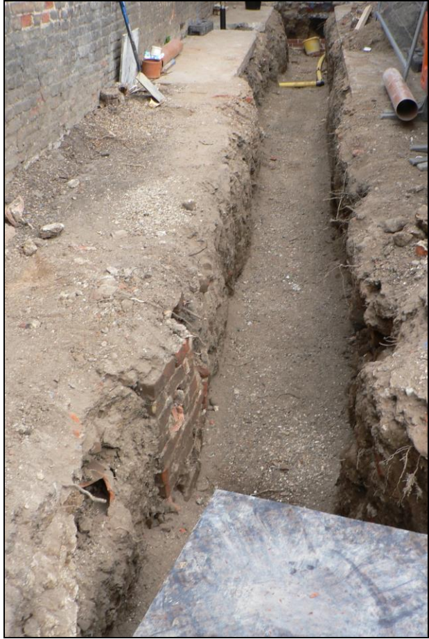
Drainage trench at rear from south
