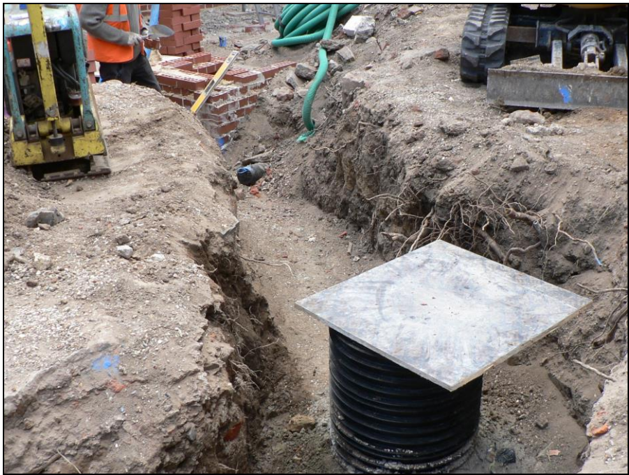
Southern end of drainage trench
