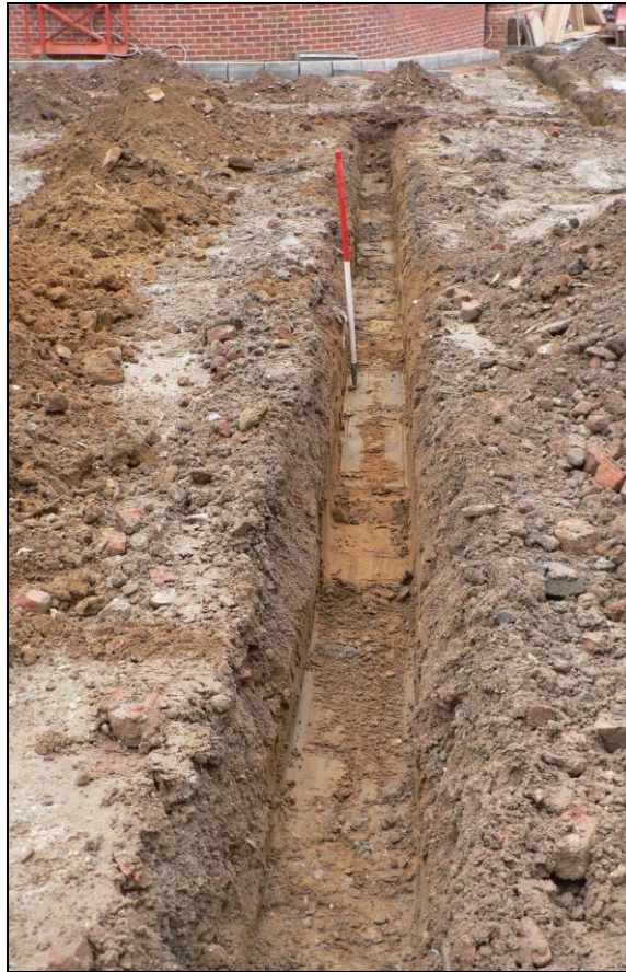
Cable trench across southern part of site towards plot 3
