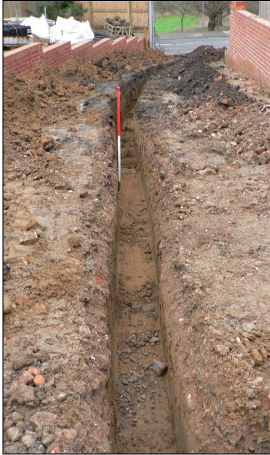
Cable trench along access road from south
