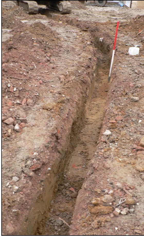
Cable trench across eastern part of site towards plot 4
