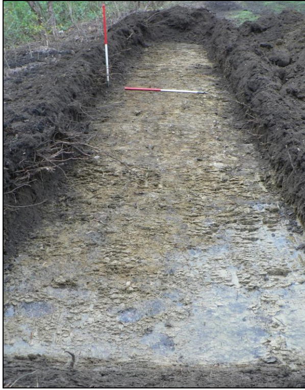
Trench 3 from west
