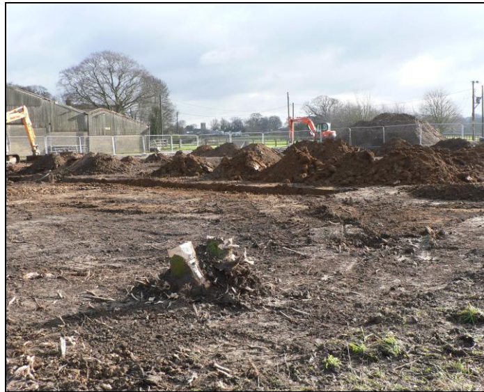
General view from northwest
