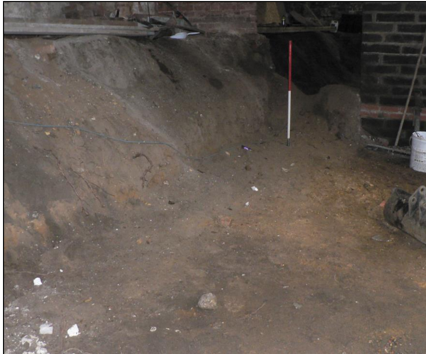
Ground reduction along southern side of building
