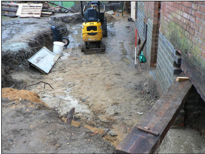
Ground reduction on southern side of building
