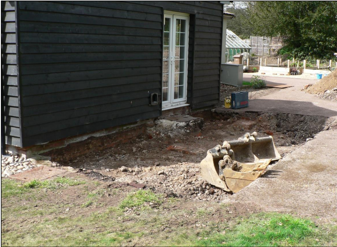
Full extent of raft foundation for northern extension
