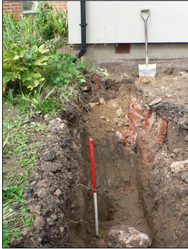
Initial trenching at southern end of eastern extension area
