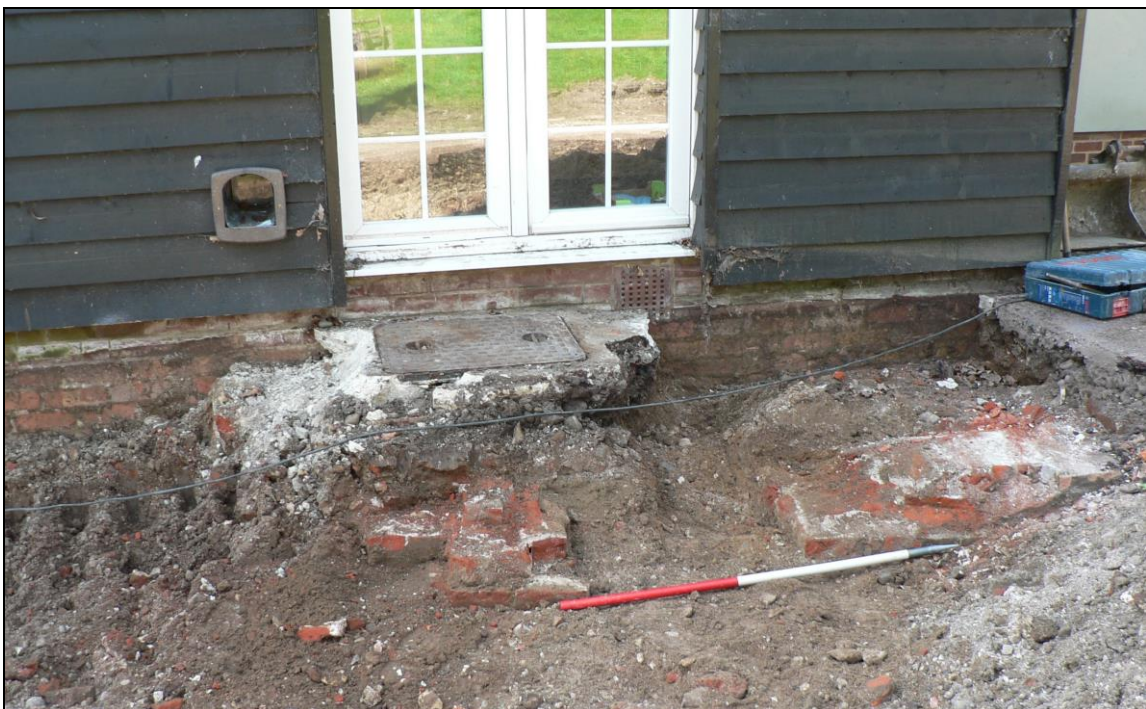
Brick foundations in southwestern corner of raft area for northern extension
