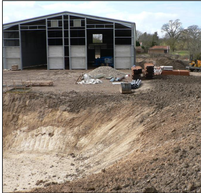
General view from east
