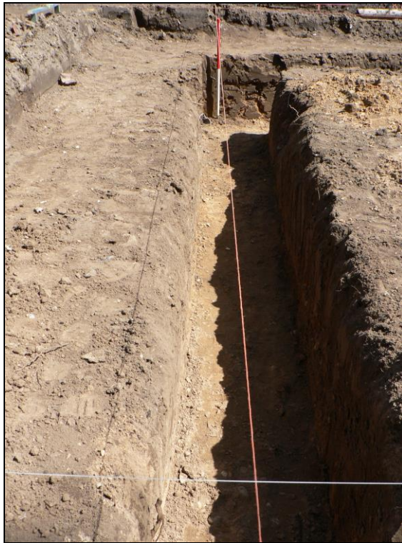
Western trench from southeast
