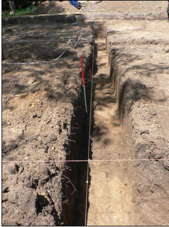
Central trench from southeast
