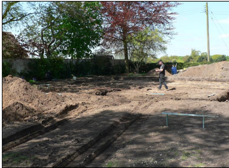
General view from southeast
