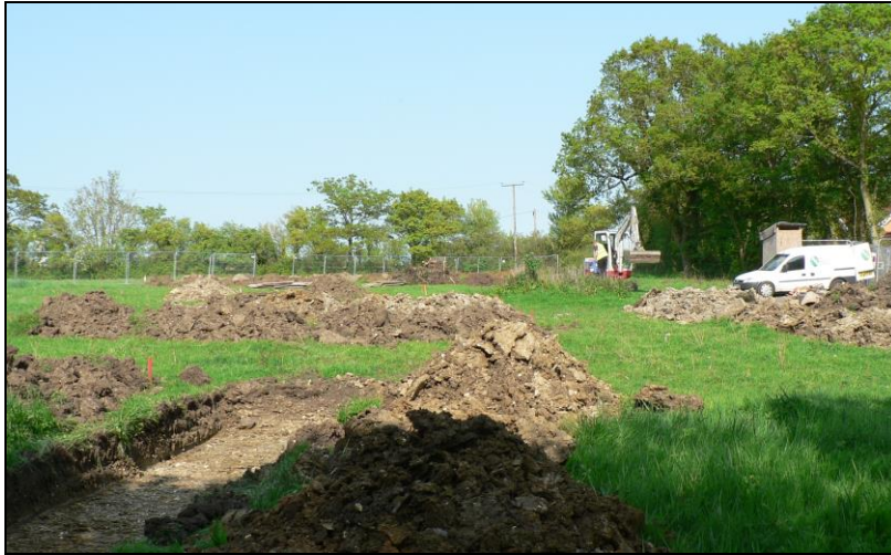
General view from west
