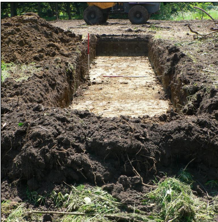
Trench 6 from northeast
