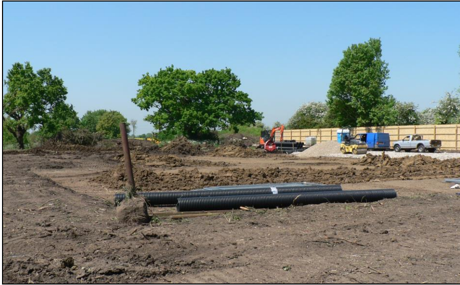
General view from southeast
