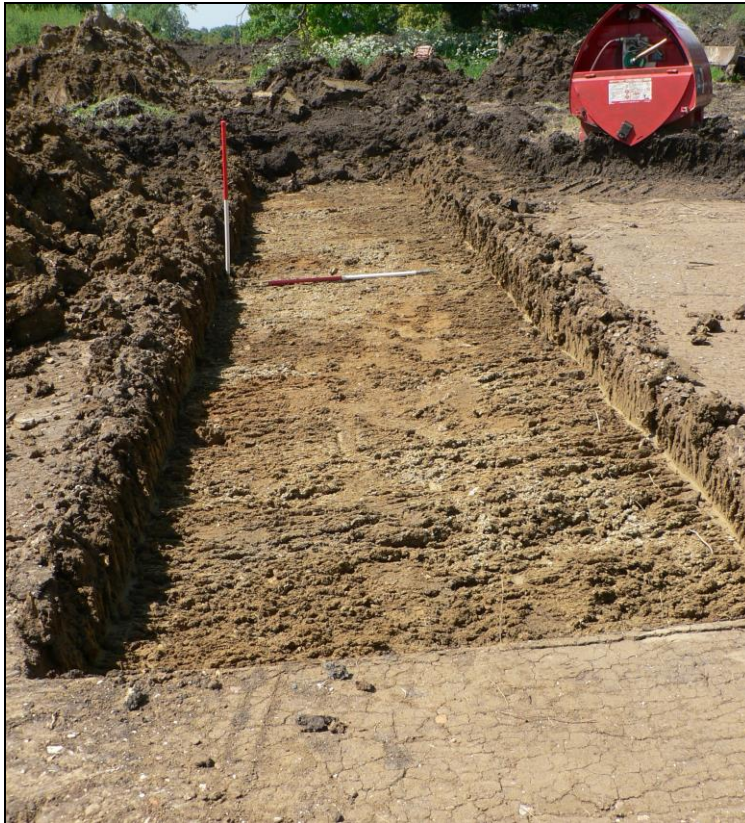
Trench 5 from southeast
