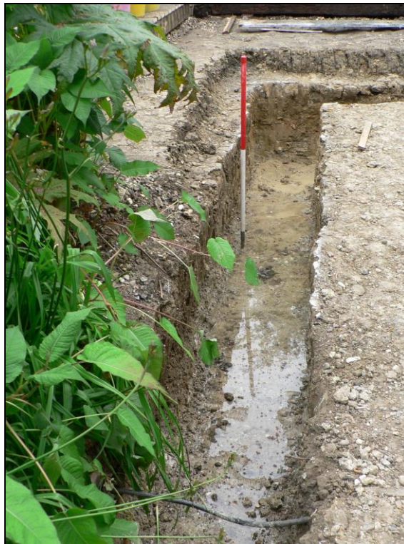
Southern foundation trench
