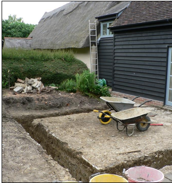
General view from southwest
