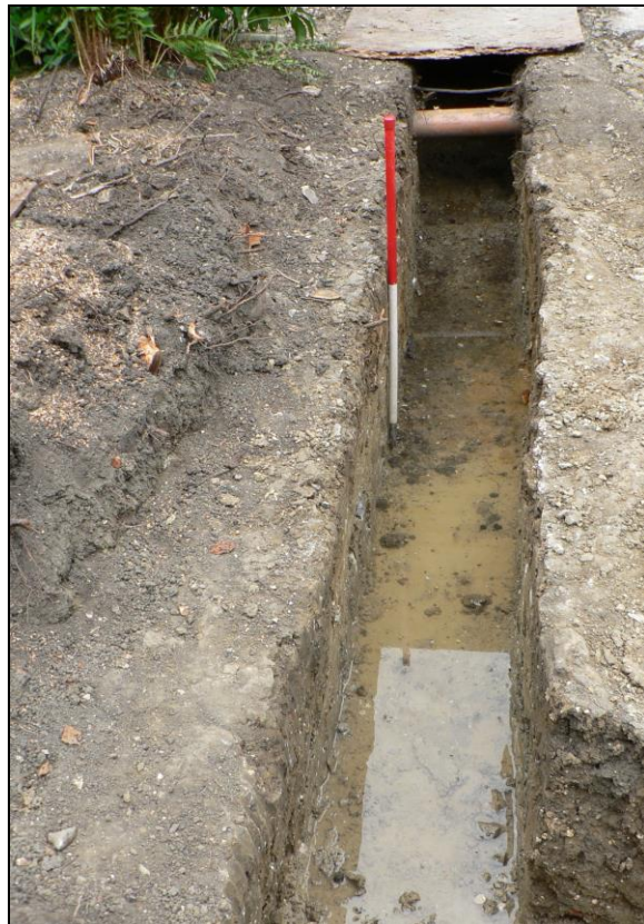
Northern foundation trench
