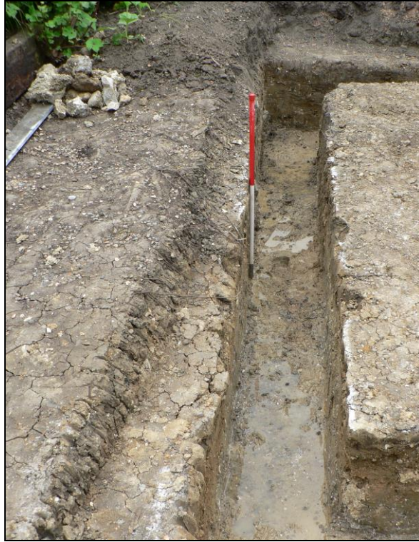
Western foundation trench
