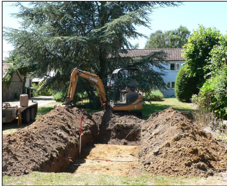
General view of trench 1 from east
