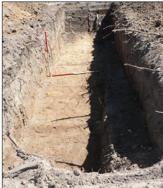
Trench 1 from southwest with pipe along southern side
