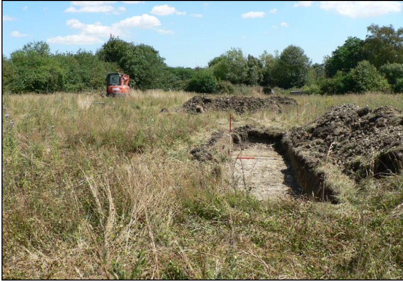
General view from west
