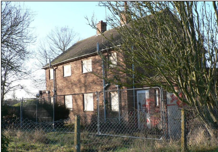
General view from northeast
