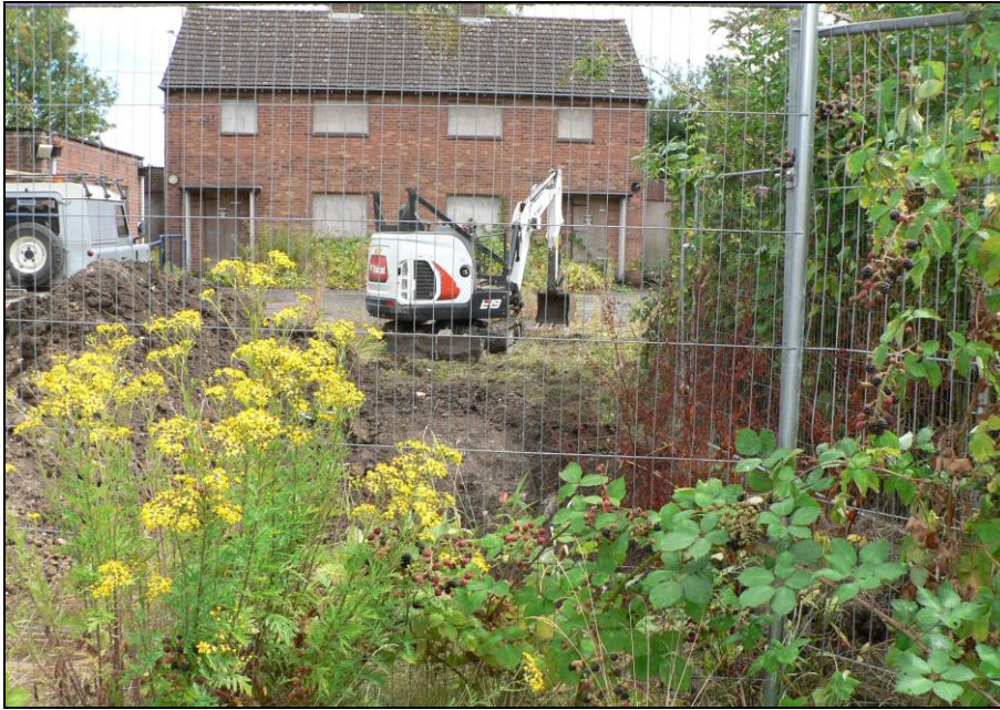
General view from west
