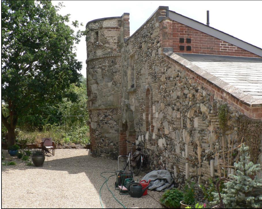
General view of eastern side of The Folly after restoration
