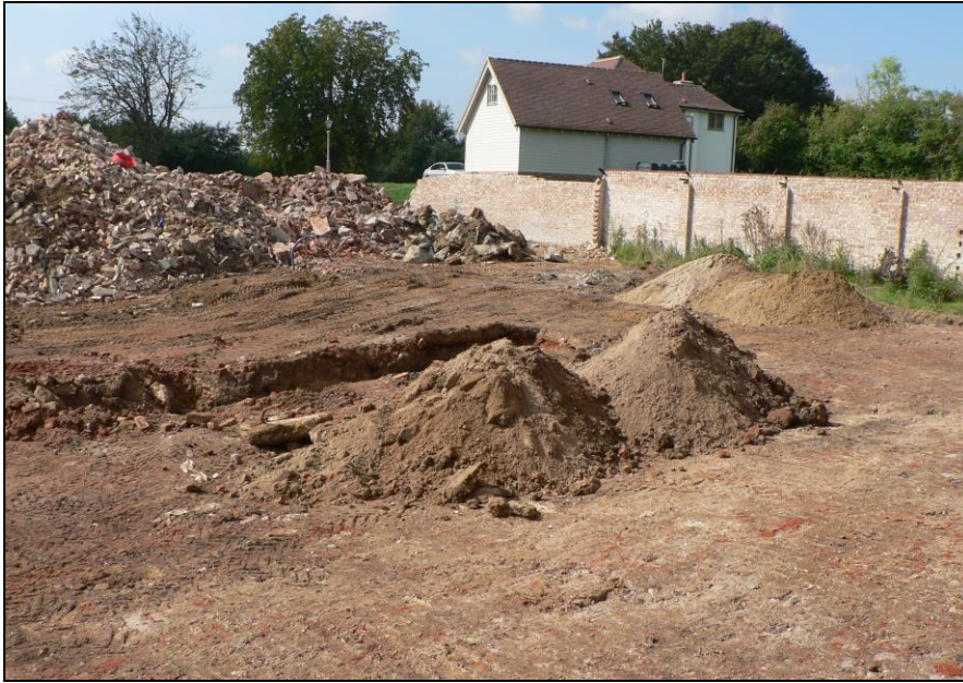
1. General view from southeast
