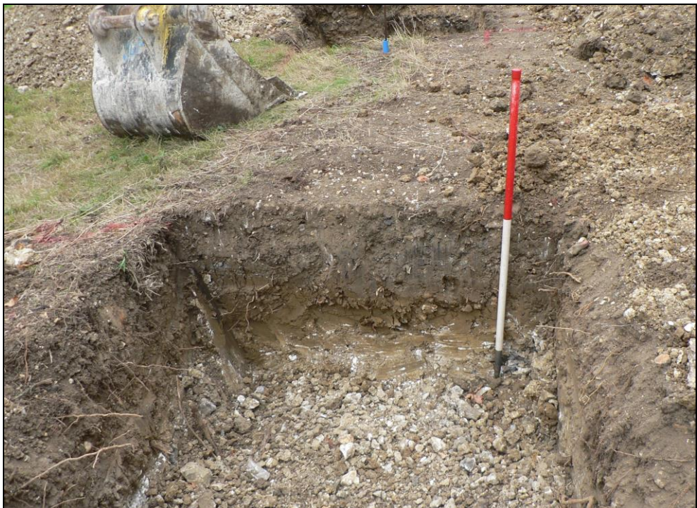
Stanchion pit on southern side of site
