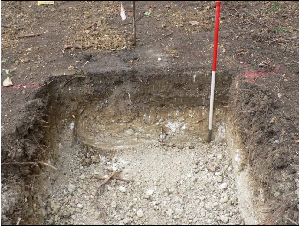
Stanchion pit on eastern side of site
