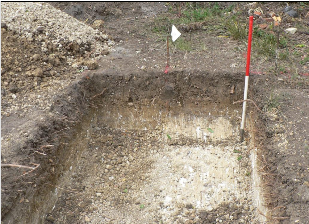
Stanchion pit on northern side of site
