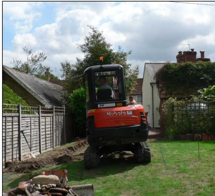
General view from north
