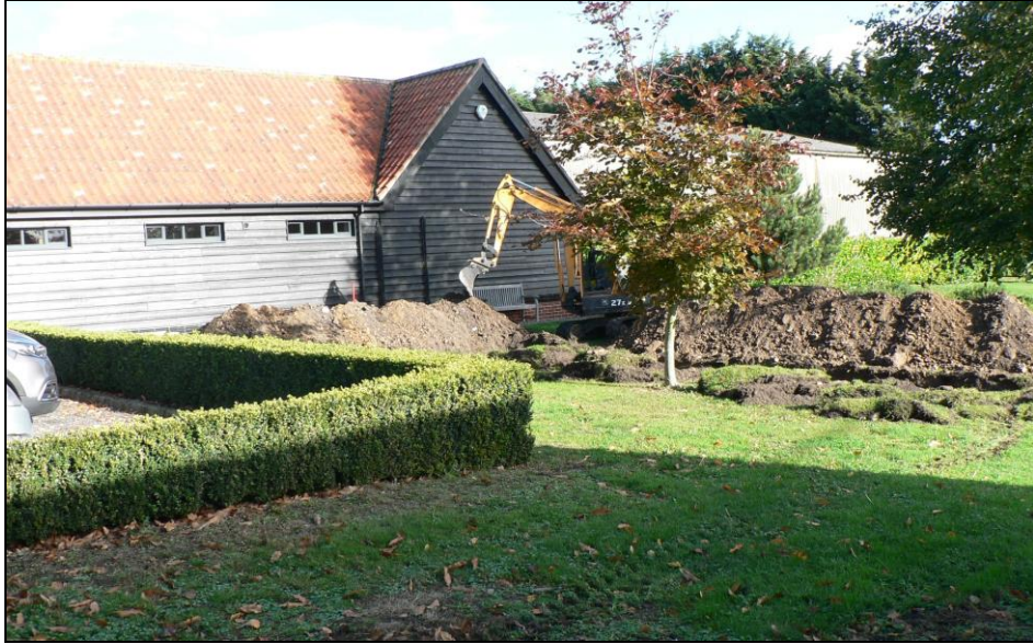
General view from southwest
