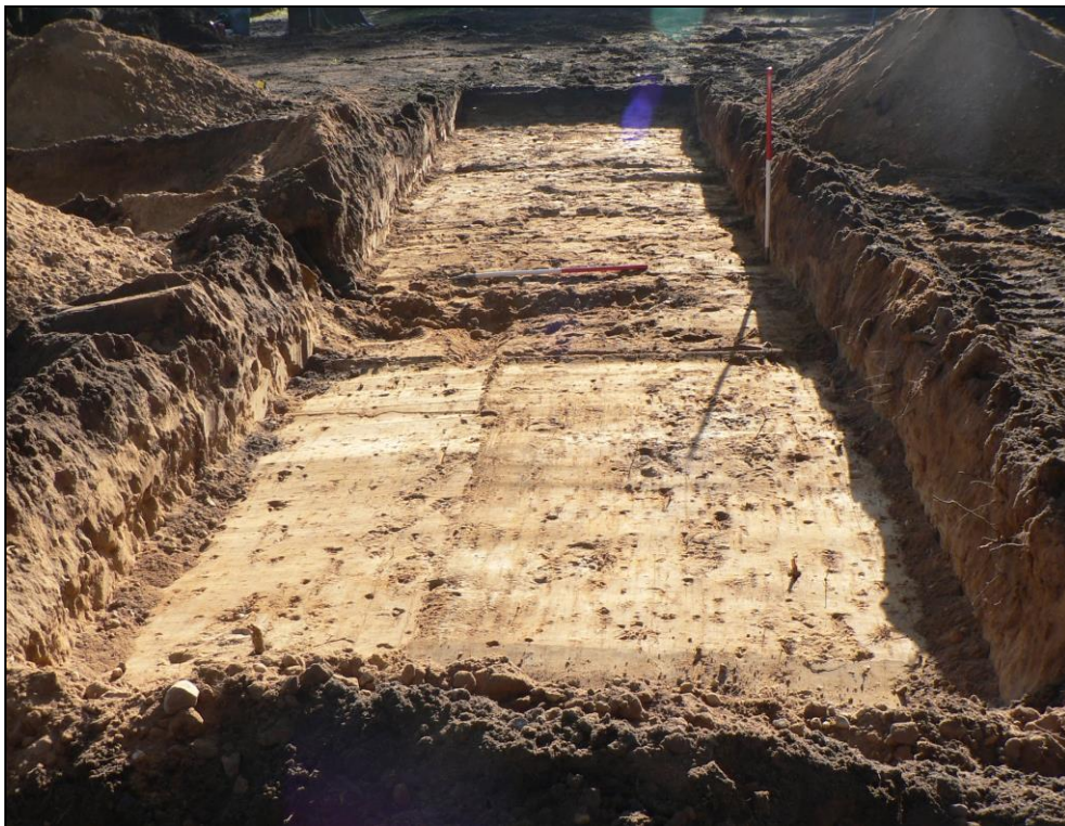
Trench 2 from southeast
