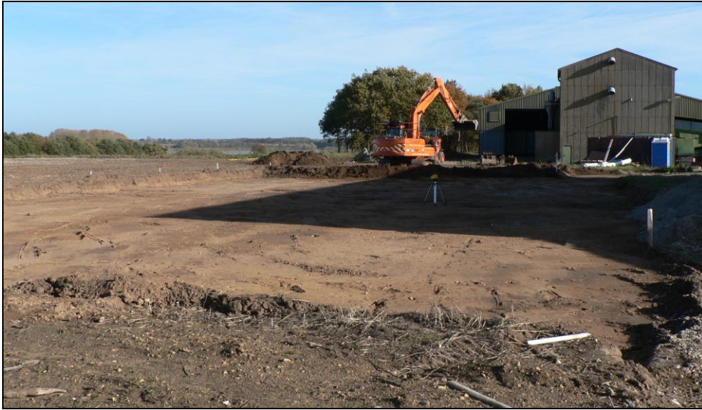
General view from southwest during soil strip
