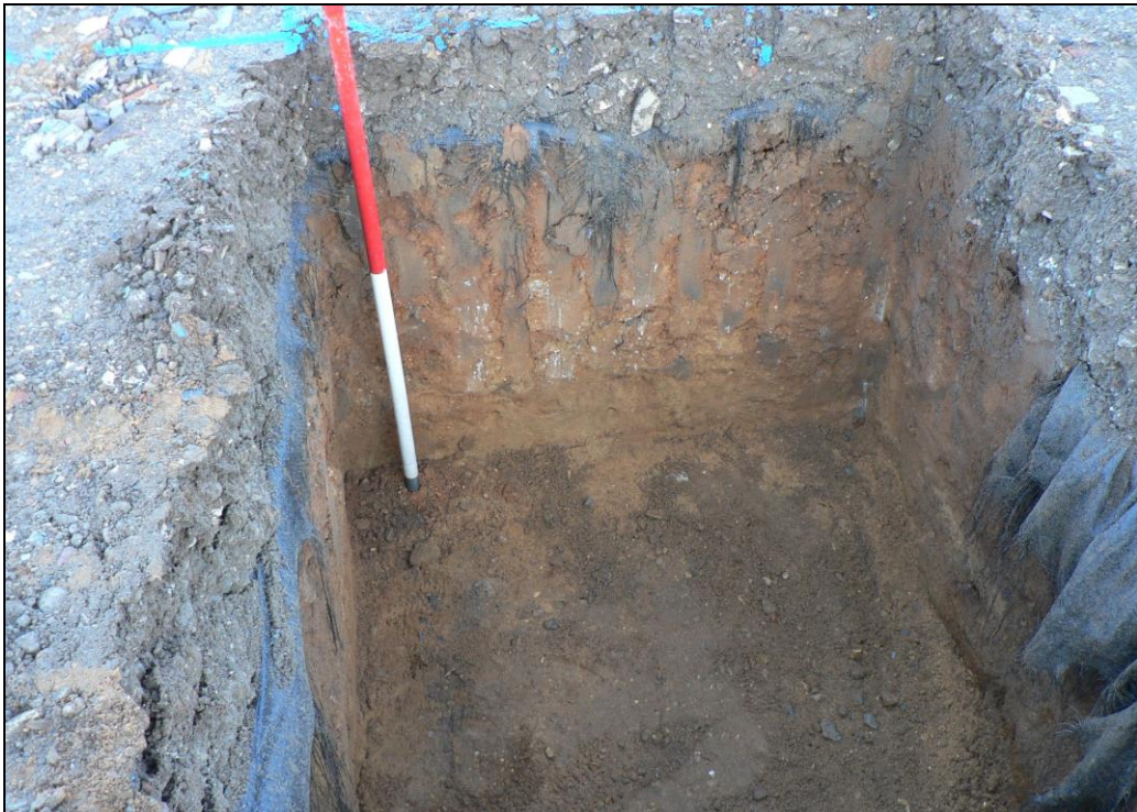
Stanchion pit on north side
