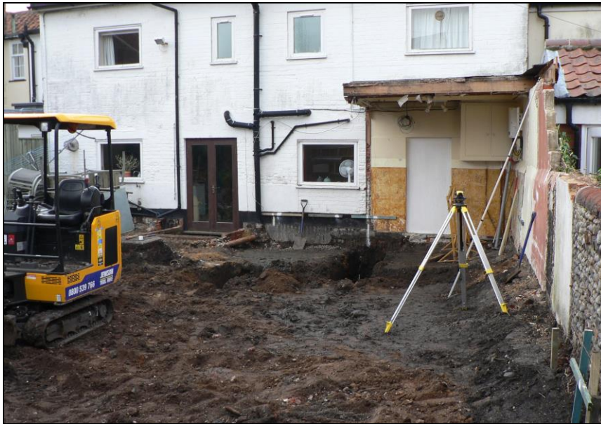
General view from north
