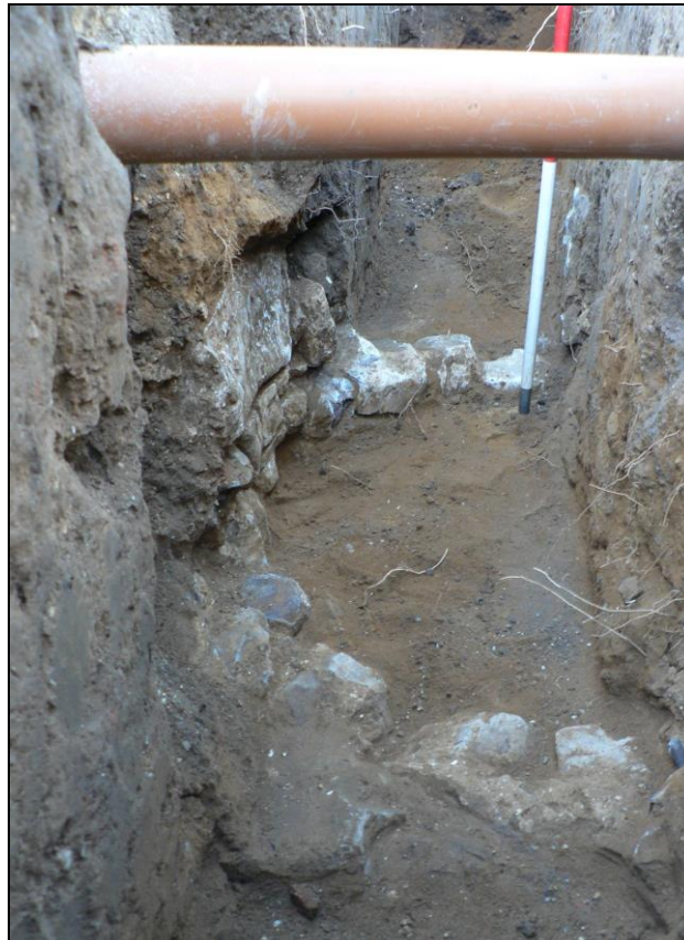
Curved wall footing 0002 from northeast
