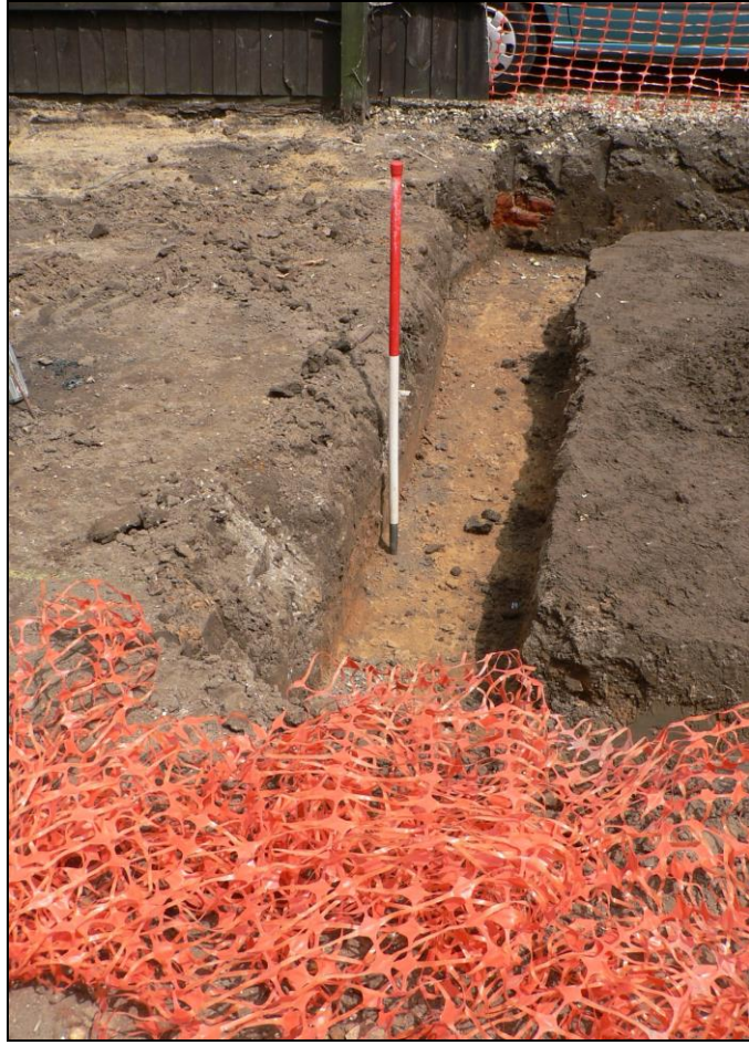
Western trench of cart lodge
