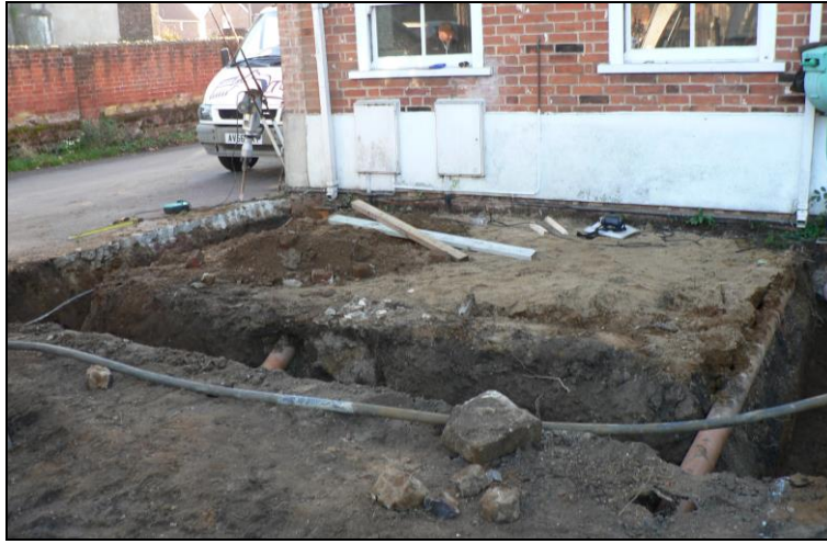
General view of extension area
