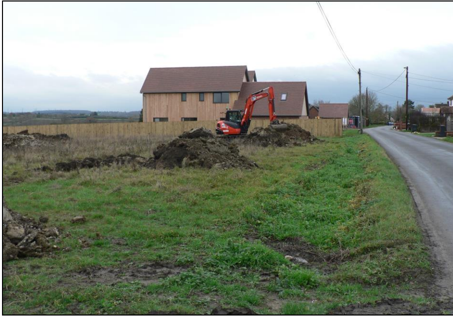
General view from northwest
