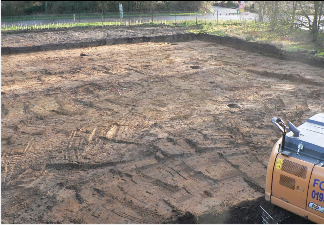
General view of excavation area from west
