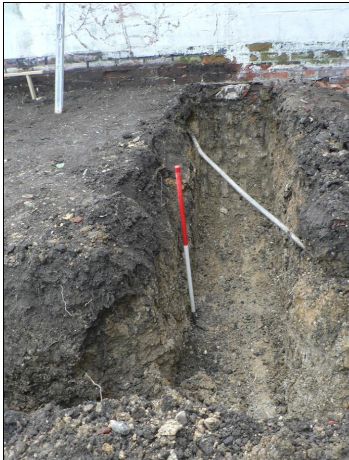
Foundation trench on eastern side
