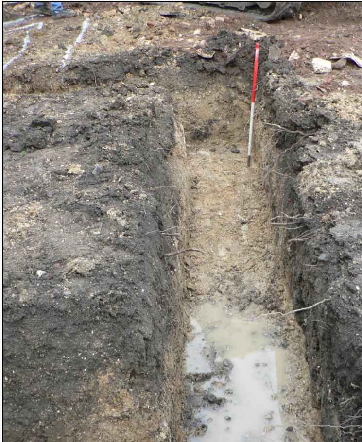
Central foundation trench from west
