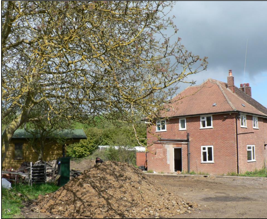
General view from southeast
