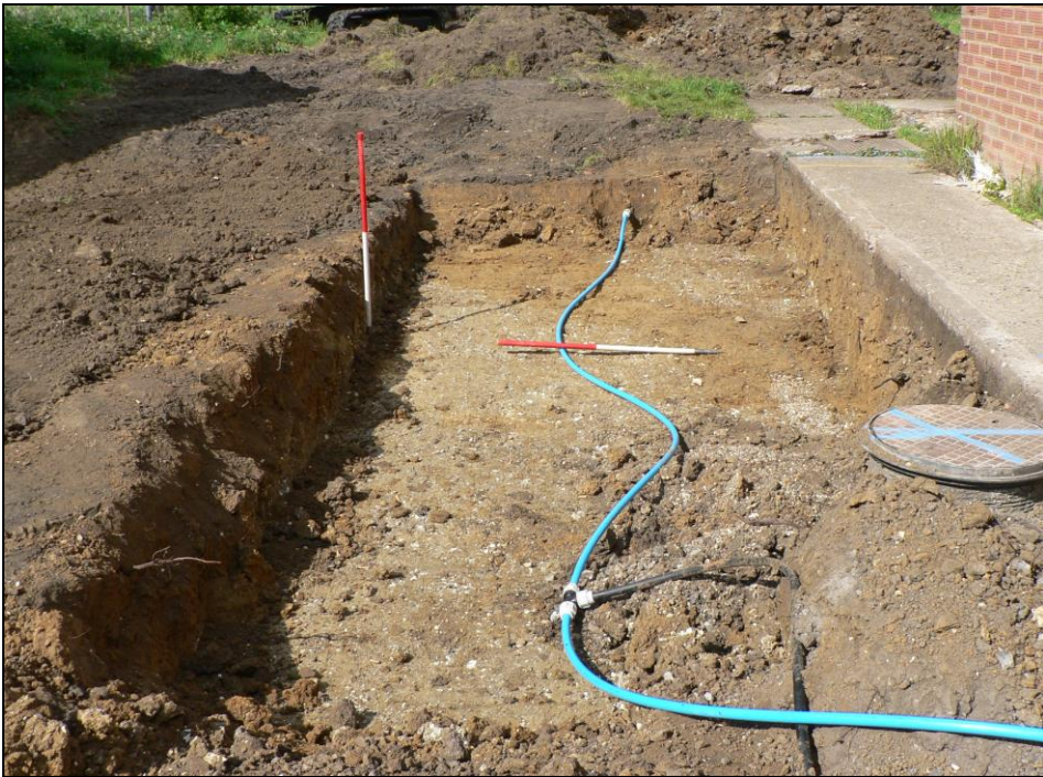
Stripped side extension area from east
