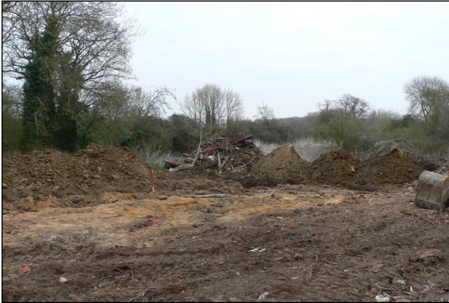
General view from southeast
