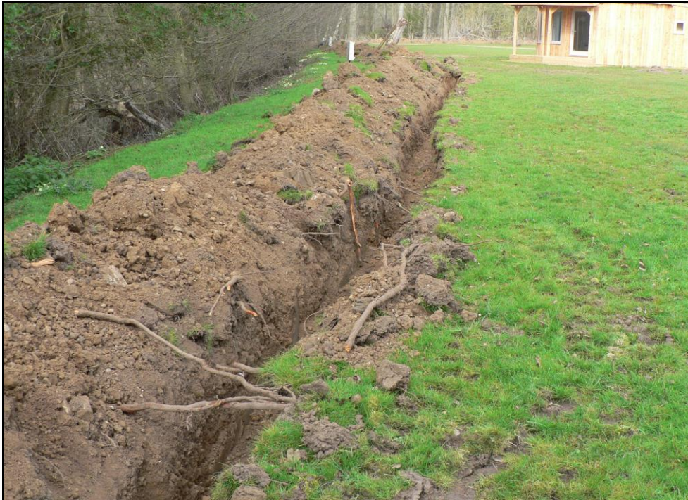
Service trench along eastern edge
