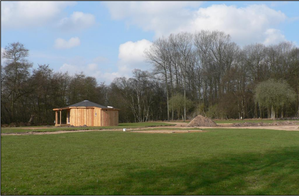
General view from north
