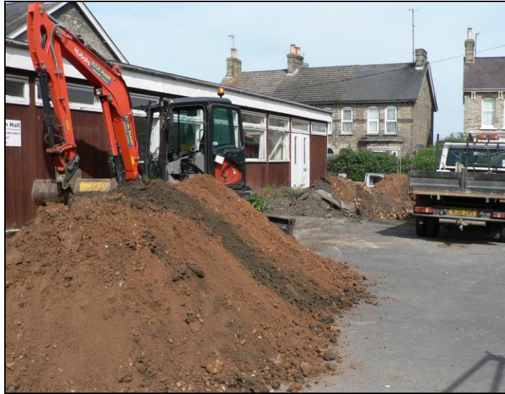
General view from southwest
