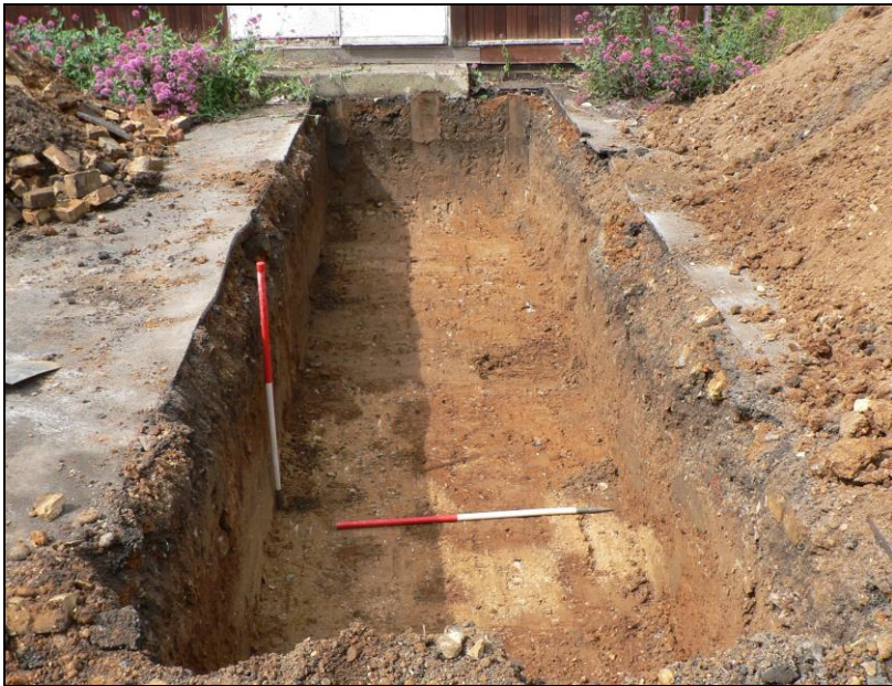
Trench 2 from west
