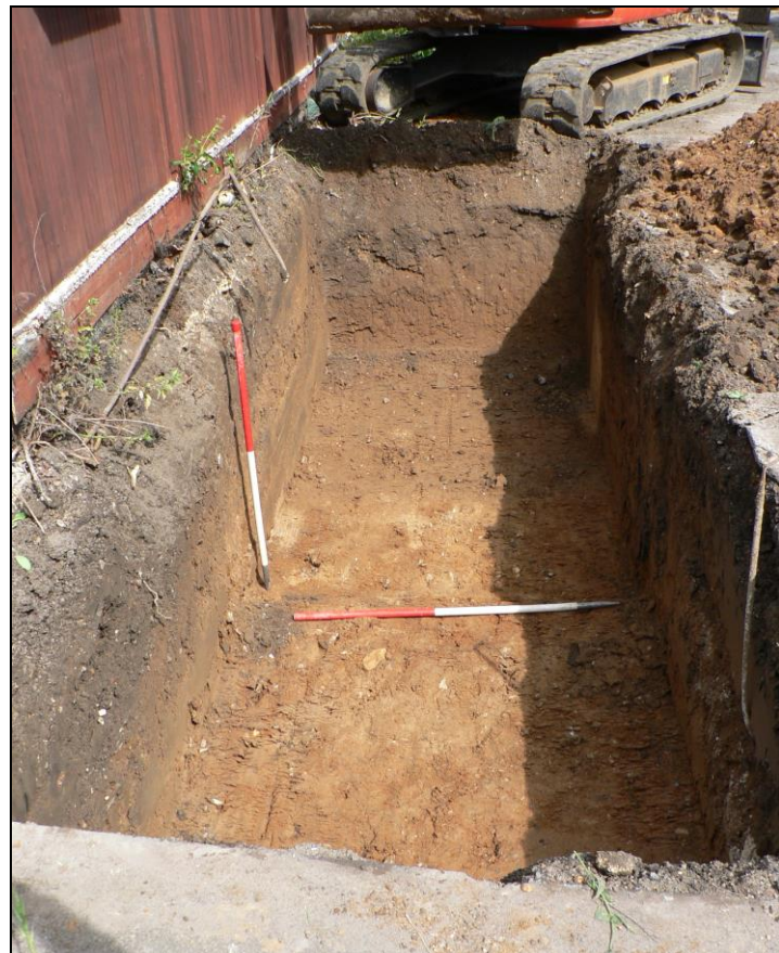
Trench 1 from south
