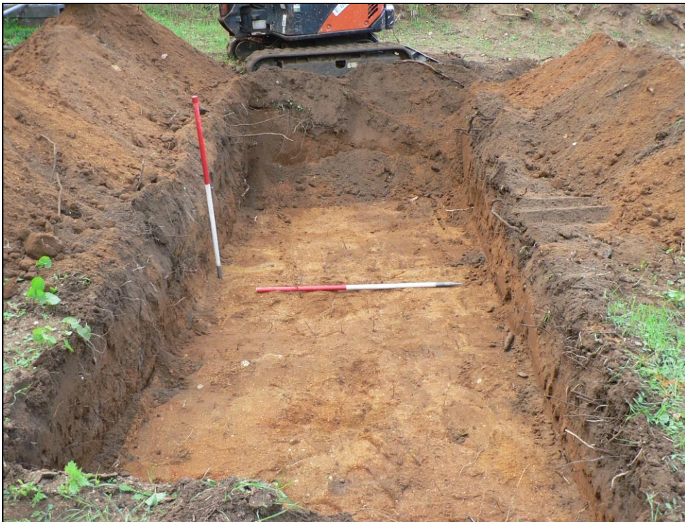
Trench 2 from east
