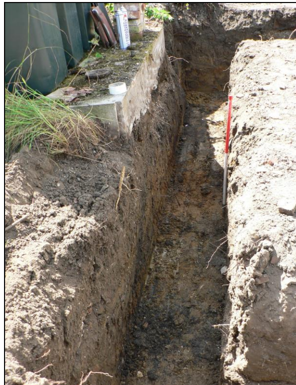
Eastern trench from north
